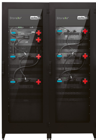
Storage Rack System SRS2028 / SRS2047
